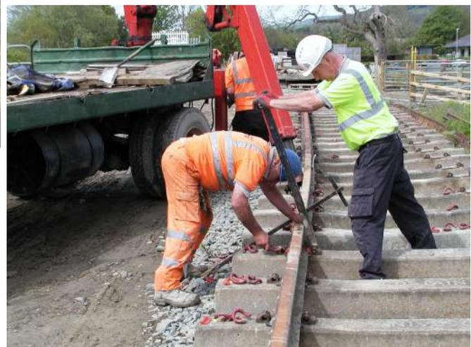
*John Mason and Peter Jump placing Pandrol clips to hold the rail in place Photo: PR*
