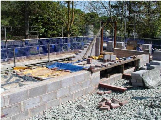
*Scaffold in place and locking room build underway. Note entrance door frame (top left) and exit slots (top right) to accommodate point rods and signal pulleys* *Photo : PR*
