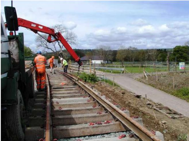
*Rail replacement whilst showing (R) the widened embankment* Photo : PR
