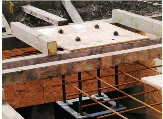
*Shuttering showing positioning of steel bolting surfaces extending below* Photo: PR
