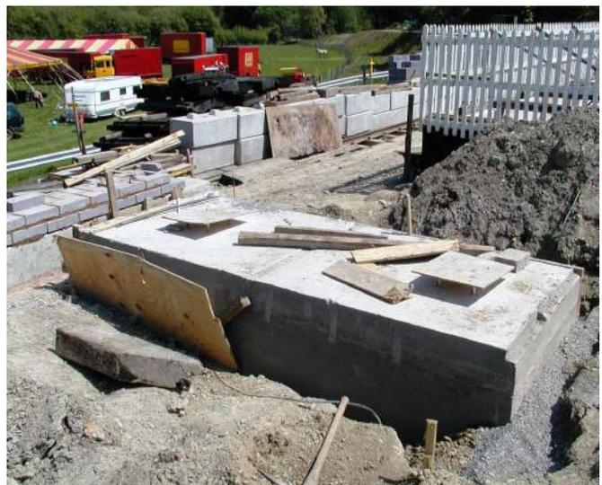
*Concrete casting complete for first pair of columns - bolting surfaces protected by plywood covers* Photo : PR
