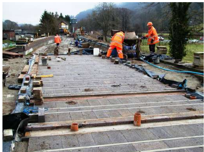
Block and beam waiting room floor nearing completion Photo: PR
