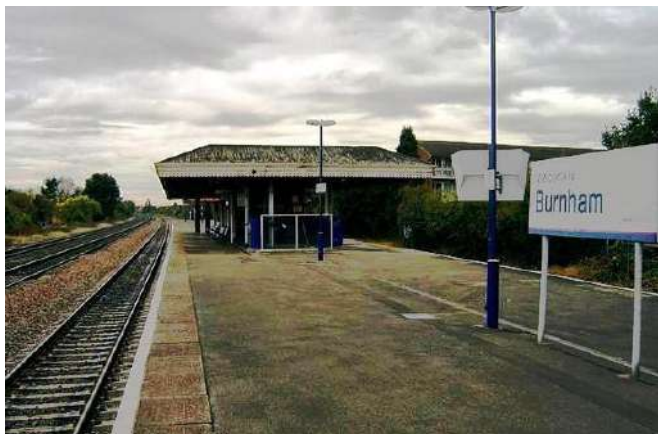
Burnham Station – with new railings Photo : Cuzza
