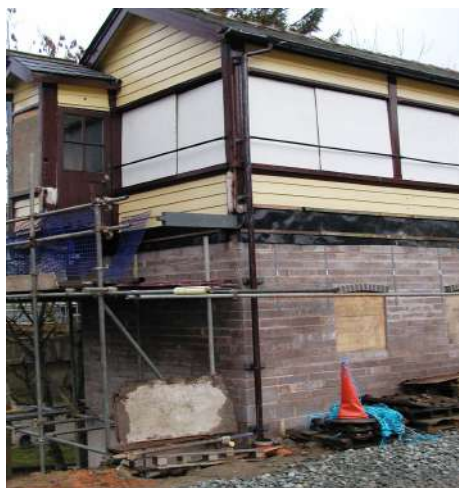
Guttering and down pipes on the signal box Photo : PR
