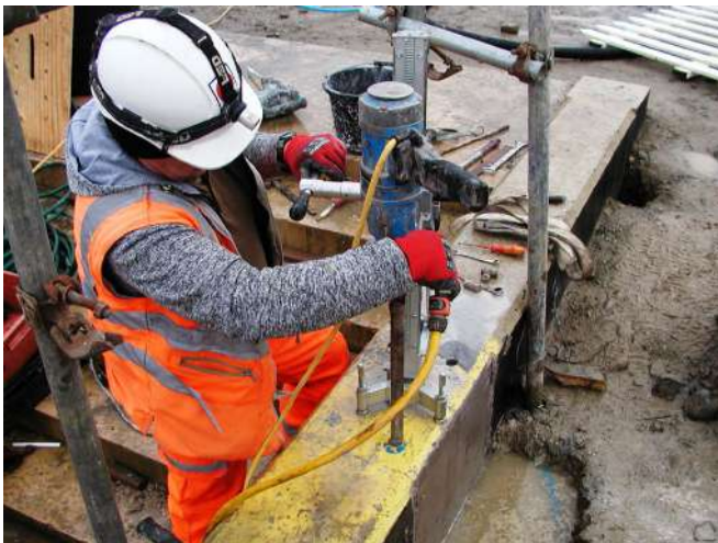
Third hole being drilled for saddle top Photo : PR
